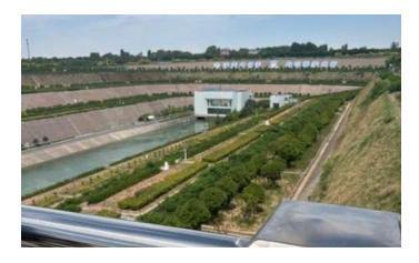
**Figure 1:** This is a part of the South-to-North Water Diversion Project. This was taken at the start of the Yellow River Crossing Project which is where the water goes underneath the Yellow River. It controls how much water is coming into the diversion project and if the water is too much, taking and giving water to the Yellow River.
