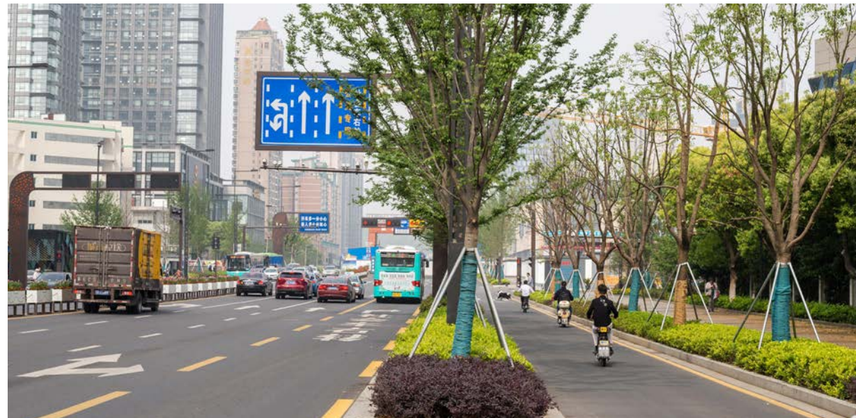
Figure 4. Median-Protected Lane for two-wheelers on arterial road in Suzhou, Jiangsu Province, China (Charles O. Cecil / Alamy Stock Photo)
